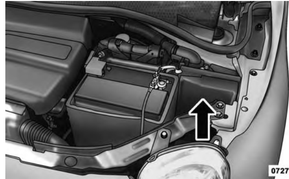
Front Distribution Unit
